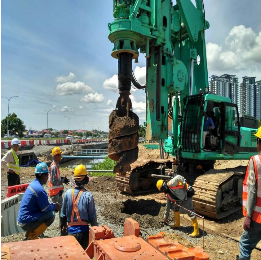
Photo 1: J5- Preliminary Test Pile:-
